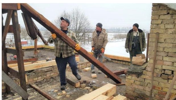
A house damaged by the war in Ukraine being repaired.
